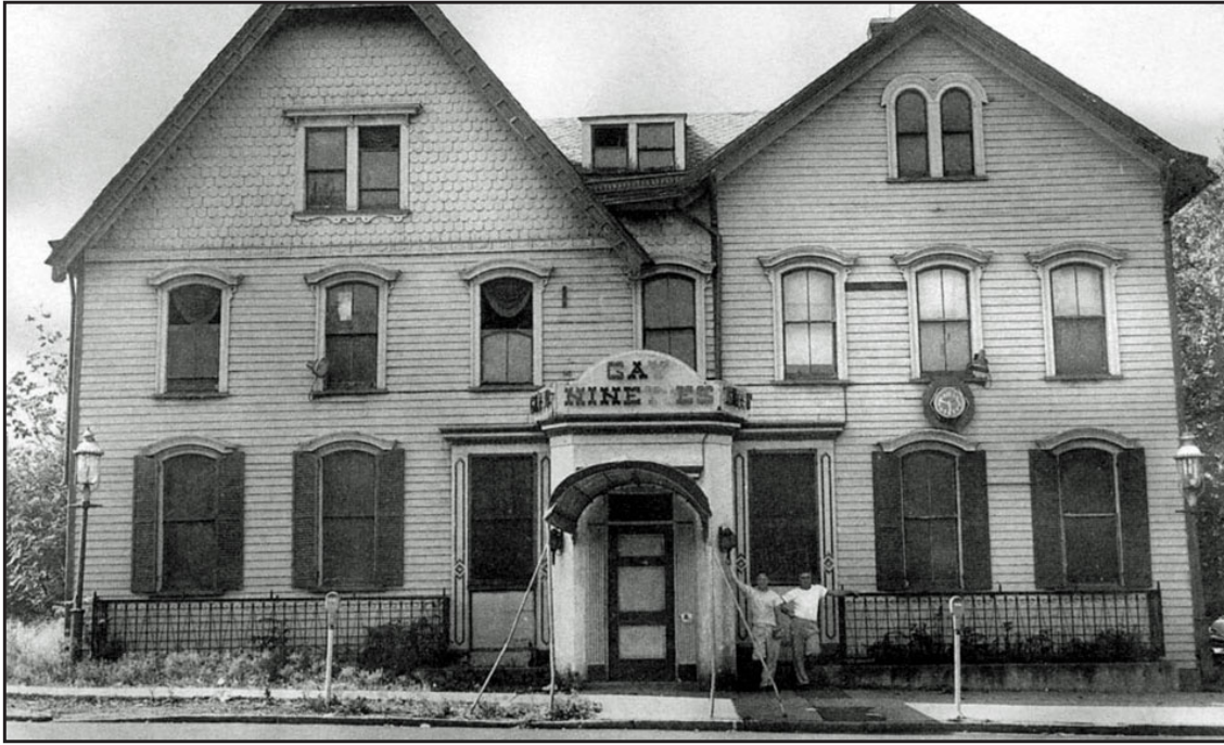
At left, Gay Nineties just before being demolished for the Garden State Parkway.
